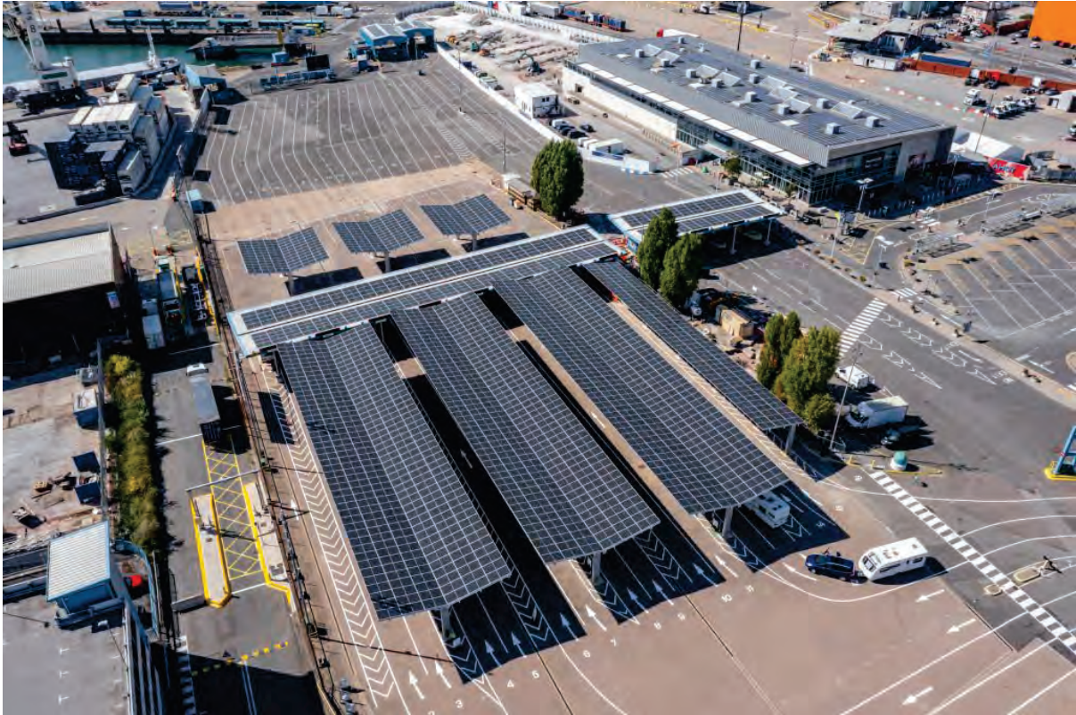
Figure 10.1: Example of solar canopy within Portsmouth International Port
